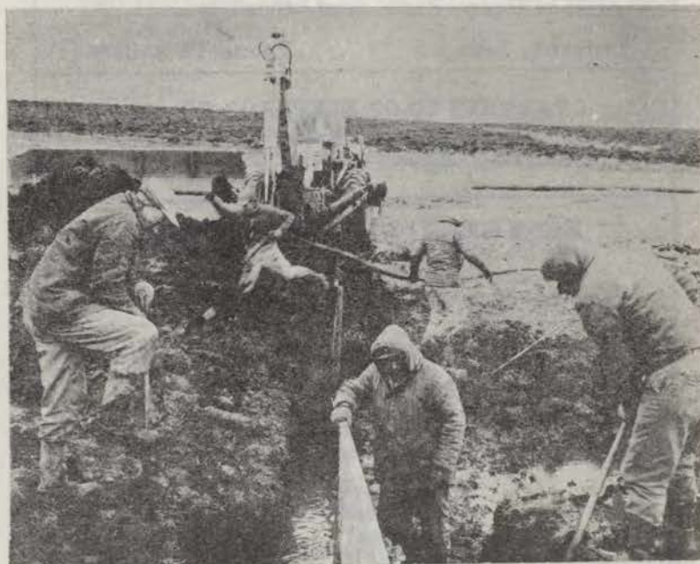
In the fall of 1965 two soil saver structures were constructed, one on the Edmund Frideres farm and the second on the Charles Dearchs farm, both of Algona.
