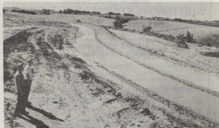
Loren Greiner, Soil Scientist, and Gerald Hollander, Area Engineer, are looking at a new type terrace, constructed this summer on the Kyle Keith farm near Algona. Note: water stored from small watershed before tile intake was installed to remove this water.
