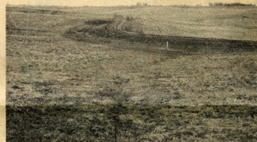
Parallel tile outlet terraces constructed on Russell Kinsinger's farm last fall.
