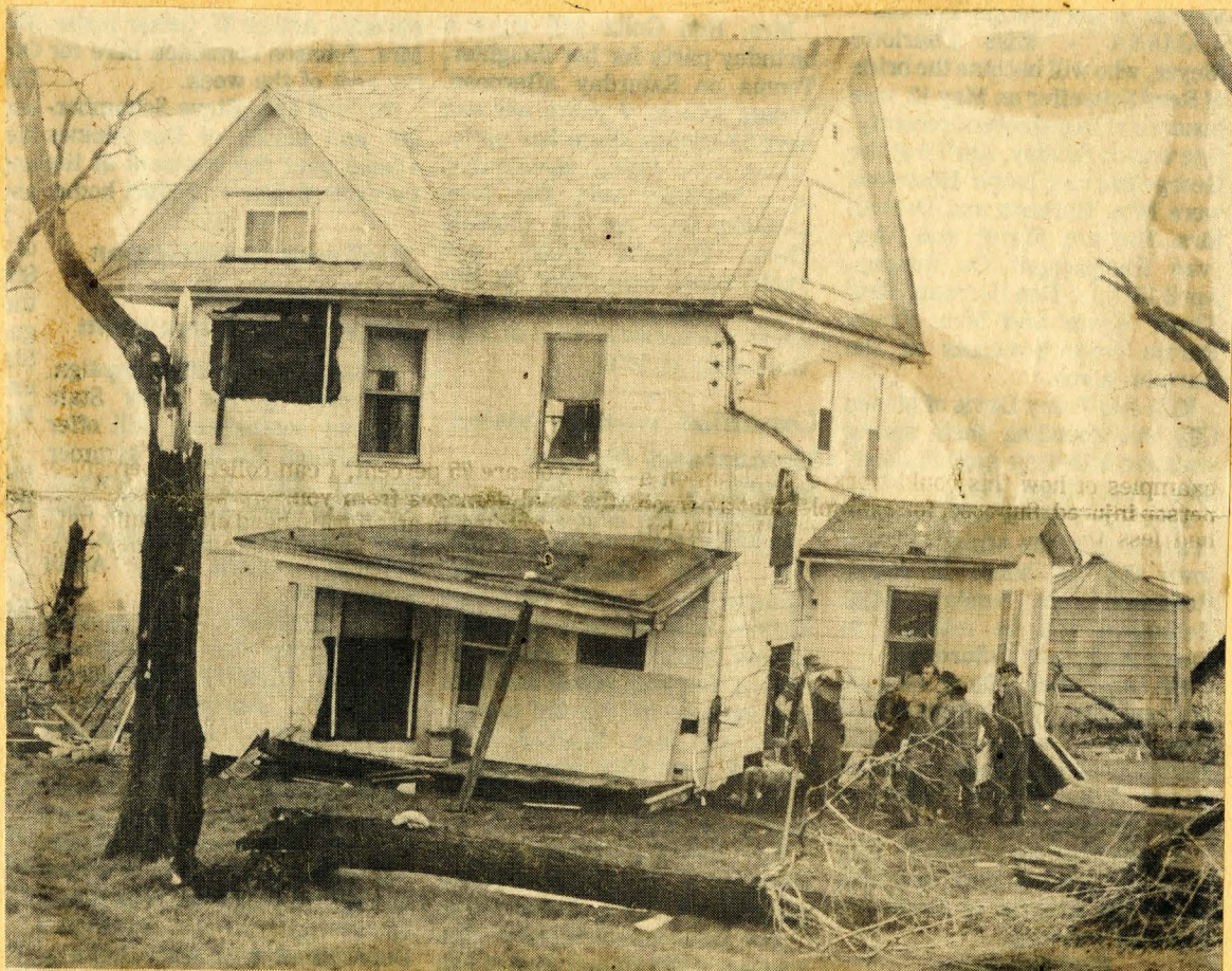
BERT O'BRIEN HOUSE WRENCHED FROM FOUNDATION House was burned Tuesday
