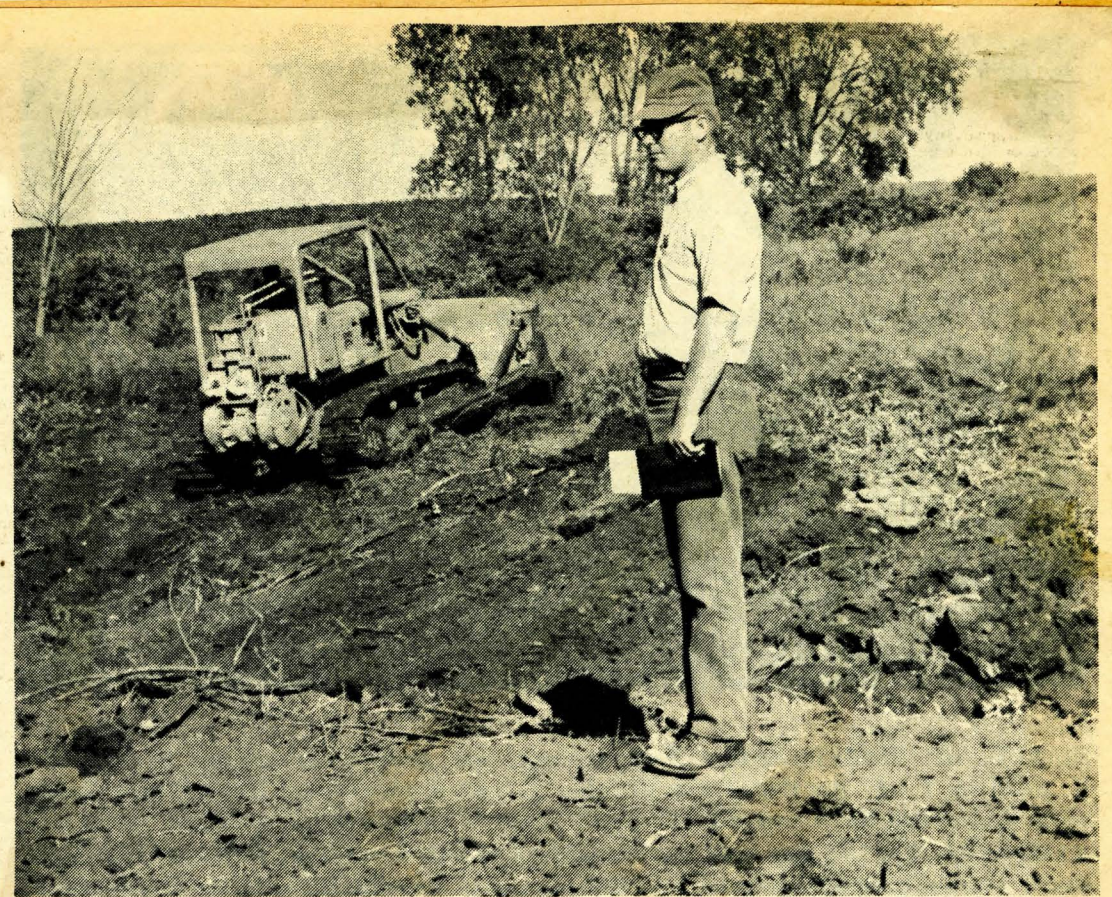
LOOKS OVER PROGRESS—Rick Cordes, Iowa County Soil Conservationist, was at the Duane Schwarting farm southwest of Homestead Friday morning as the Gahring Construction Company, Williamsburg, did the grading necessary for a grade stabilization structure being built. Cordes was standing where the earth dam would come in from the south. In back of him is another ditch going north which will be controlled by the work being done. A six and one half foot diameter tube will go through the dam east and west to control both ditches. Tile, 3400 feet of it, will also go up both sides of the ditch.
