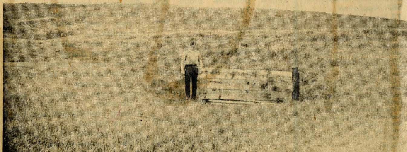
DOEHRMANN BUILDS EROSION CONTROL DAM — Allan Doehrmann, Williamsburg, has built an erosion control dam and a grass waterway on his farm north of Williamsburg. He said he was losing too much subsoil through erosion and noted
