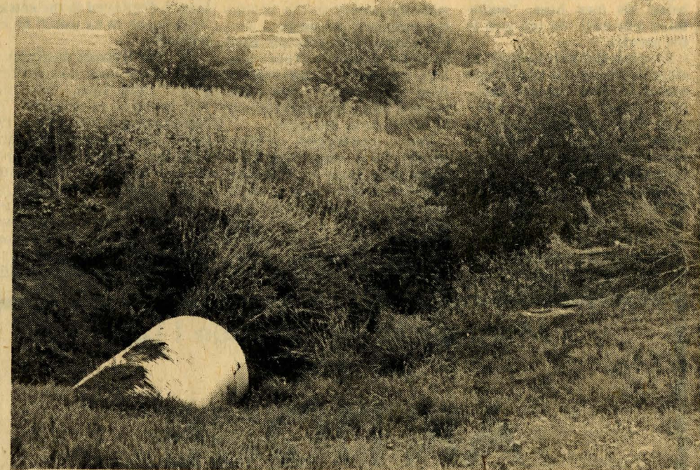
DIRECTED TOWARD CREEK — Water gathered by erosion control dam on Allan Doehrmann's farm is channeled toward Old Man's creek by pipe extending through dam. Doehrmann is one of five farmers in county who have signed long-term contracts with federal government for conservation work. They have agreed to do all
