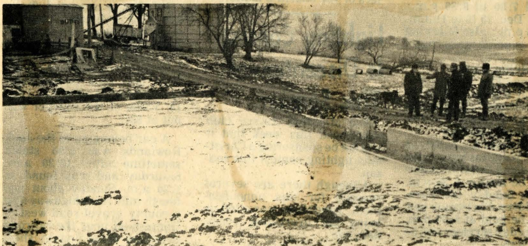
LOOKS AT MANURE PIT —ASC and SCS committees toured the Nyle Felling farm southwest of Marengo. Cattle manure pit in foreground was frozen at time of tour. Project has not been approved because not enough reinforcement steel was used to meet specifications set by the state and federal governments for this type of cost sharing project. The SCS does not design manure pits. All concrete pits either meet specifications according to plans already on file or plans drawn up must be certified by a licensed engineer as meeting specifications. Runoff from the concrete manure pit here will go into lagoon across the road in back of the men looking over the project. Left to right are Lambert Elwood, Fred White, Carl Lantz, Felling, and Lowell McKean, county extension director.
