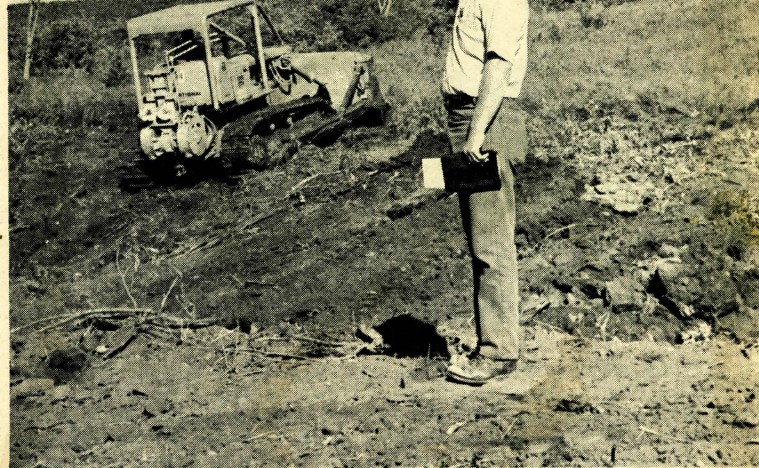
LOOKS OVER PROGRESS—Rick Cordes, Iowa County Soil Conservationist, was at the Duane Schwarting farm southwest of Homestead Friday morning as the Gahring Construction Company, Williamsburg, did the grading necessary for a grade stabilization structure being built. Cordes was standing where the earth dam would come in from the south. In back of him is another ditch going north which will be controlled by the work being done. A six and one half foot diameter tube will go through the dam east and west to control both ditches. Tile, 3400 feet of it, will also go up both sides of the ditch.
