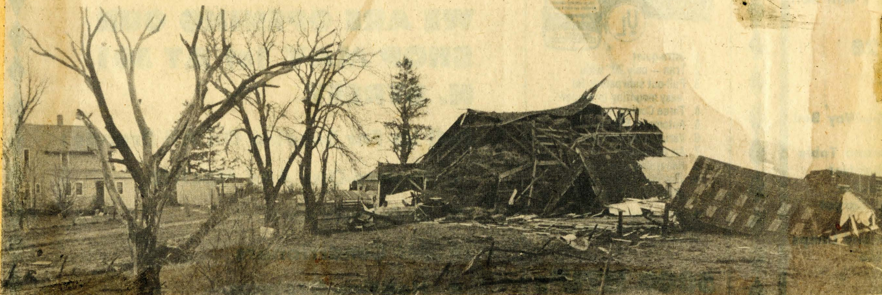
ALL OUTBUILDINGS WERE DESTROYED ON THE JAMES TAYLOR FARM
