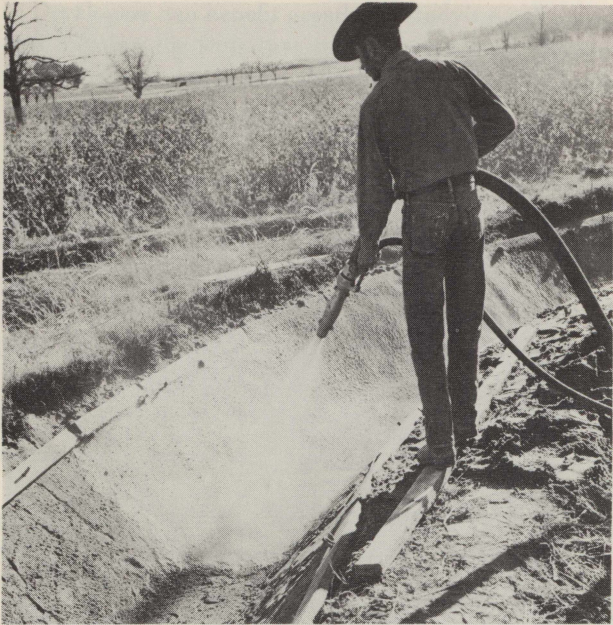
A farmer sprays concrete into a new irrigation ditch. Without this lining, some soils take in so much water that very little reaches its planned destination.
