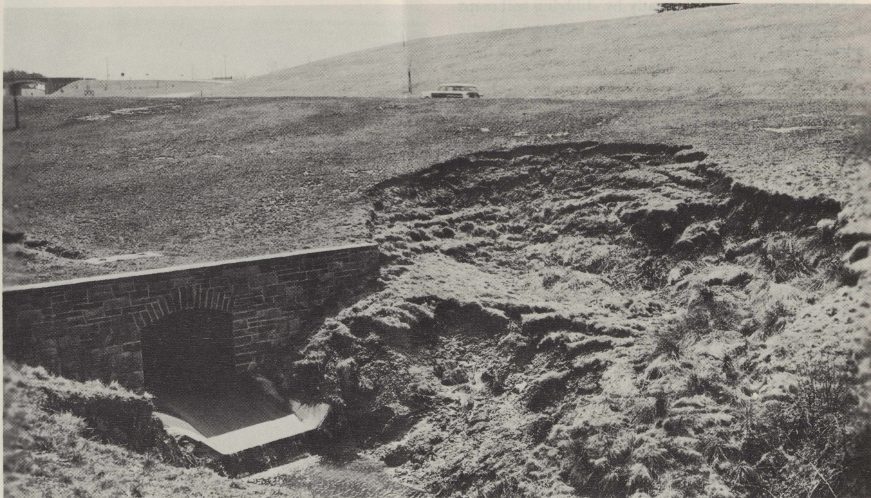
Concentration of water causes some soil to slip. The alternatives are to make the slope more gentle or to divert water from the hillside above.
