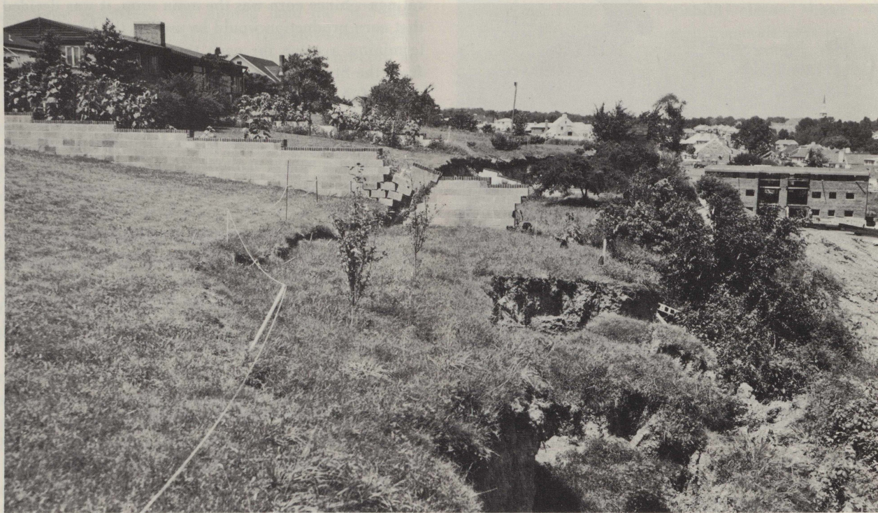
BUREAU OF PUBLIC ROADS Builders of the apartments on the right cut back the hillside too steeply, causing the unstable, gravelly soil to slip and cave in.
