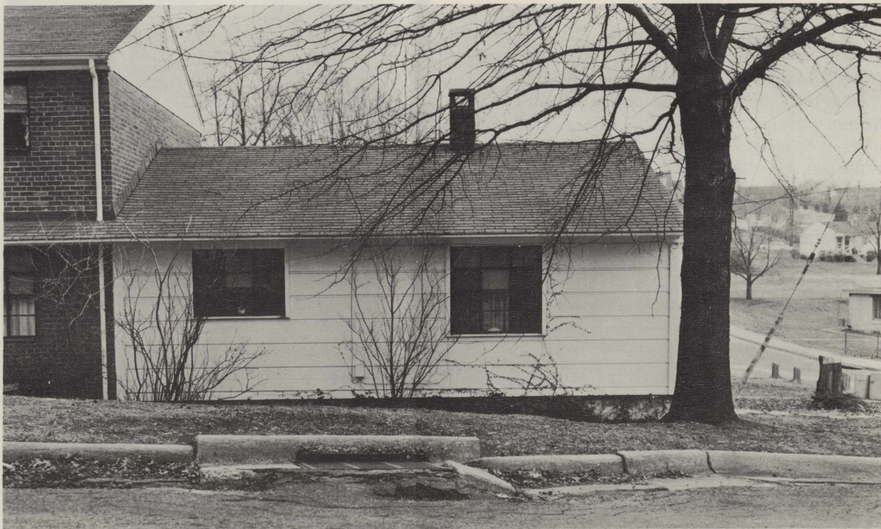
Shrinking of the soil underneath this gutter is due to the tree's absorption of water. The only solution is to remove the tree. Soil surveys can tell prospective builders about such problems.
