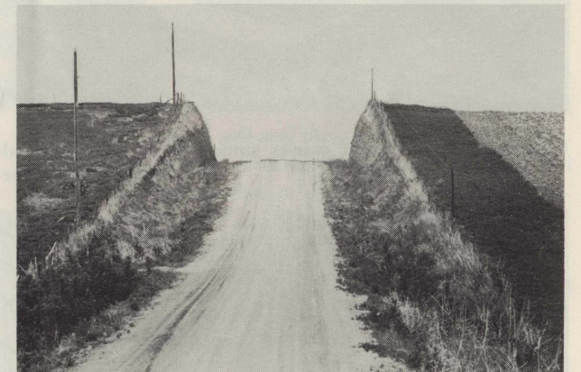
IOWA HIGHWAY COMMISSION I-14-11 Cutbanks are almost vertical in the fine-grained loess soil of the Midwest. Most soils cave in if sloped at such a severe angle.
