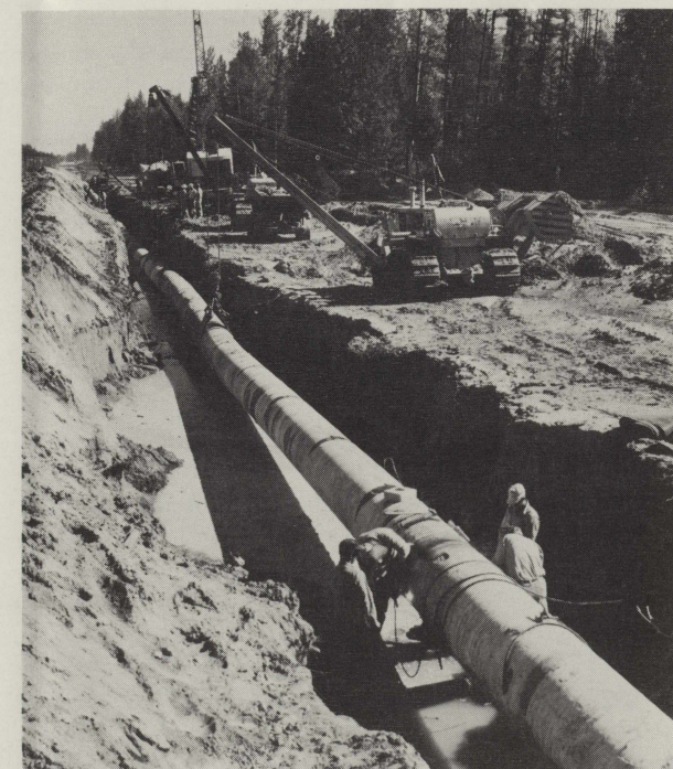
When oil and gas companies dig ditches for laying pipelines, soil information is helpful in preventing corrosion of the pipes and erosion of the soil.
