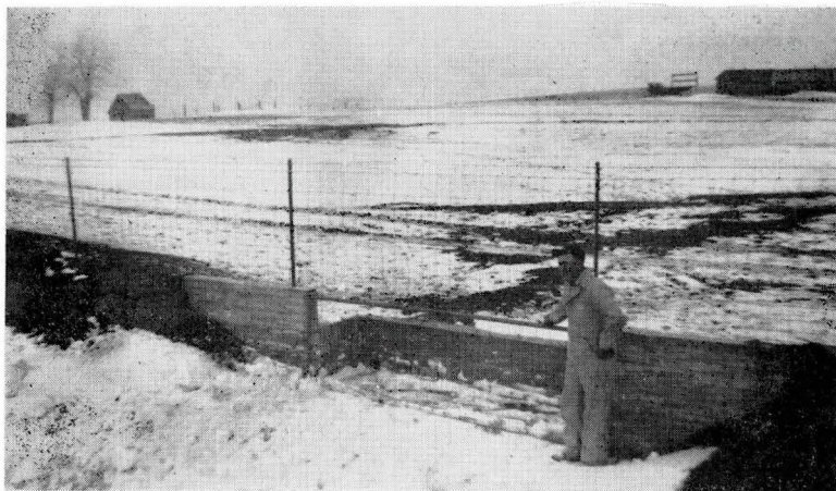
Curtis Darbyshire, by one of his tile outlet and erosion control structures.
