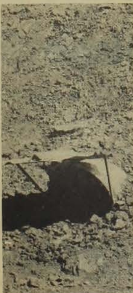
Left below—12" hooded outlet high on the pond.
