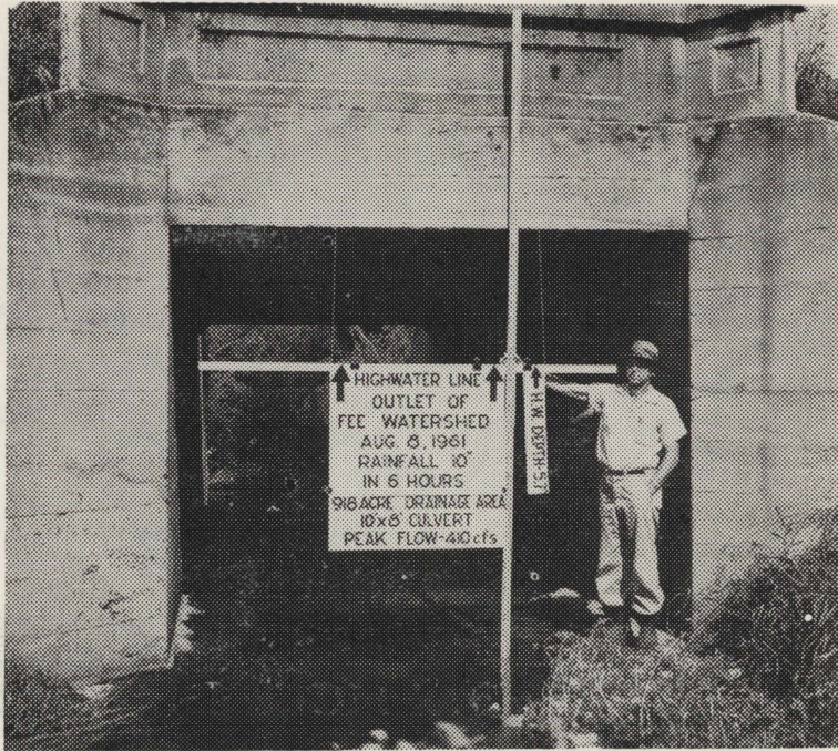
"This Culvert did not run full"
