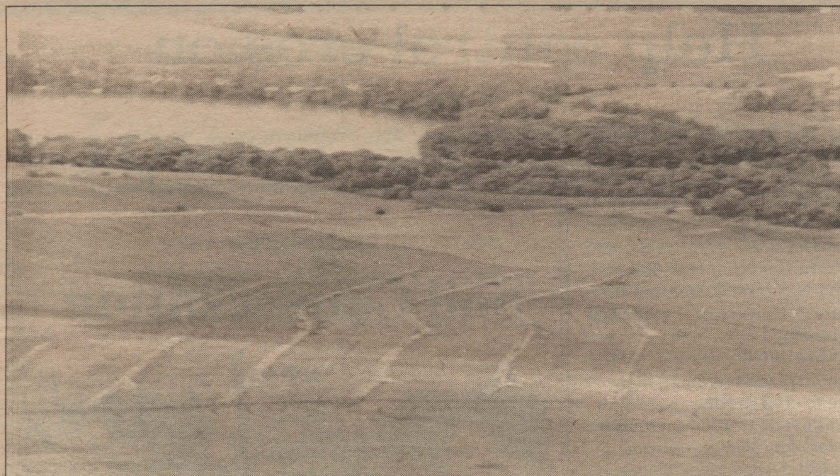
Don Schubert, south of Spirit Lake. Six parallel tile outlet grassed backslope terraces.
