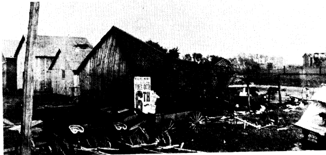
tornado." The storm struck about 8 p.m. In the countryside, barns were overturned and destroyed, and fruit
