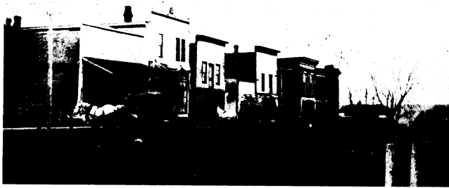
West side of Main Street looking north
