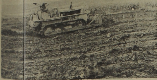
SHAPING WATERWAY --Bob Ruser, Ida Grove contractor, is pictured shaping a waterway on the Dutler Farm just south of Ida Grove.
