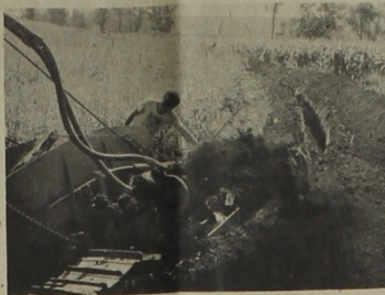
TILING --The working-end of the tiling machine puts out a lot of dirt. Here a Lunzman Trenching crew installs drainage tile on the Kenny Bower farm south of Battle Creek. Field supervisor is Ken Palm, assisted by David Bolles and Ferd Boger of Ida Grove. Over 21 miles of tile were installed in Ida County last year.
