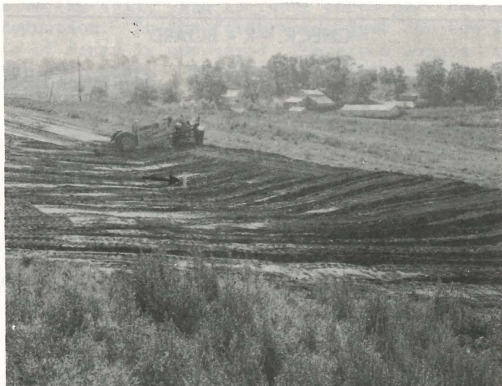
Construction of the terrace is nearly completed here. The arrow points out the intake pipe for the underground outlets. Roy L. Yoder & Sons were contractors on the job for both earth-work and tiling.
