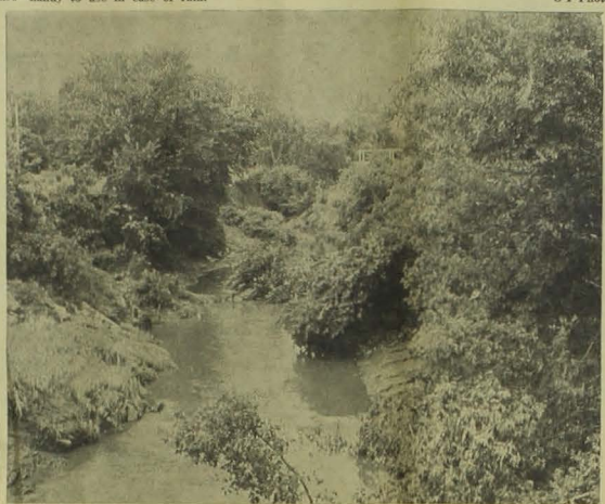
Debris from last week's high water has clogged Keg Creek through Glenwood. Tree limbs, sometimes entire trees, telephone poles and other rubble are shown in this photo, taken from the Green Street bridge.
