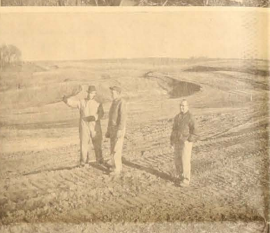
CLEVE AND BILL BENNETT—have long felt the erosion control was an important consideration in a good farming operation. To provide the best possible control, the Bennetts, started on a terrace building project on their farm in Pleasant Valley Township. The Bennetts are shown above installing one of the intake pipes used. The completed job is shown with Howard Bayle, SCS, explaining to Cleve Bennett the best method of farming the terrace while Merle Fender looks on. Fender, SCS technician from Eldorado, designed and laid out the Bennett terrace system.
