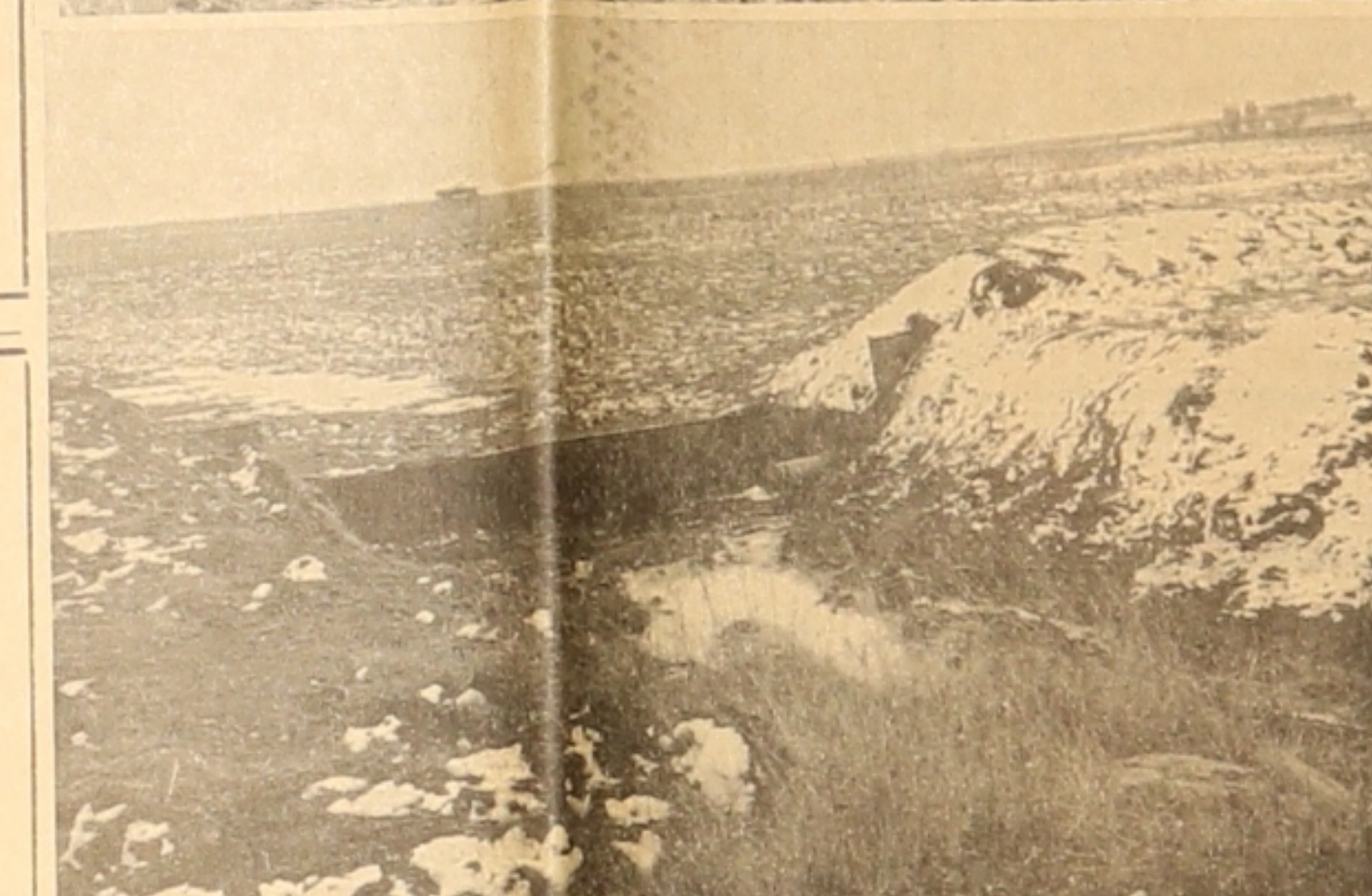
USING A GLASS-COATED—tee wall structure to stabilize the lower end, Virgil Pickar was able to build a grassed waterway on his farm in Bethel Township. The structure also provides an improved tile outlet.
