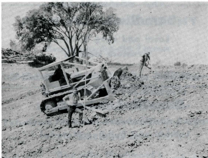
This pond was built by Jerry Miller in Franklin Township. LaVerne Lucas holding the rod and Jacobs on the Instrument are checking it out. Bouge and Walker construction contractor from New London is putting the final touches to the fill.
