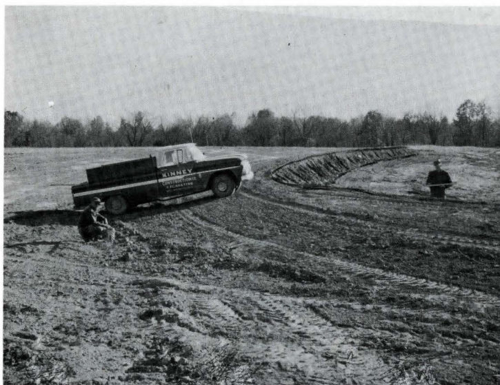
One of three parallel, cut and fill, seeded backslope terraces built by Buck LaMar in Union Township. These terraces reduce ground slope between terraces so are most useful on the more rolling ground. Tile inlets were installed to carry off surface water. This allowed all ditches and waterways to be done away with.
