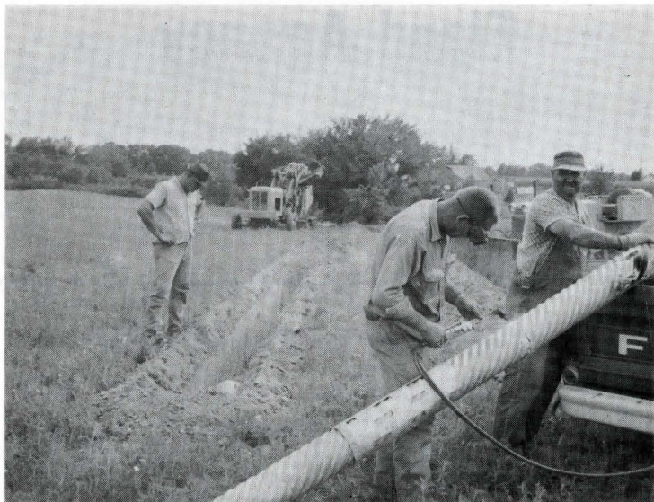
Tile inlet Terraces - Bob Zaiser is looking at one of his tile inlets being installed by Ken Springsteen, tiler from Morning Sun. Terraces were later constructed using these inlets to take water from the terraces. Tile inlet terraces are the ultimate in erosion control.
