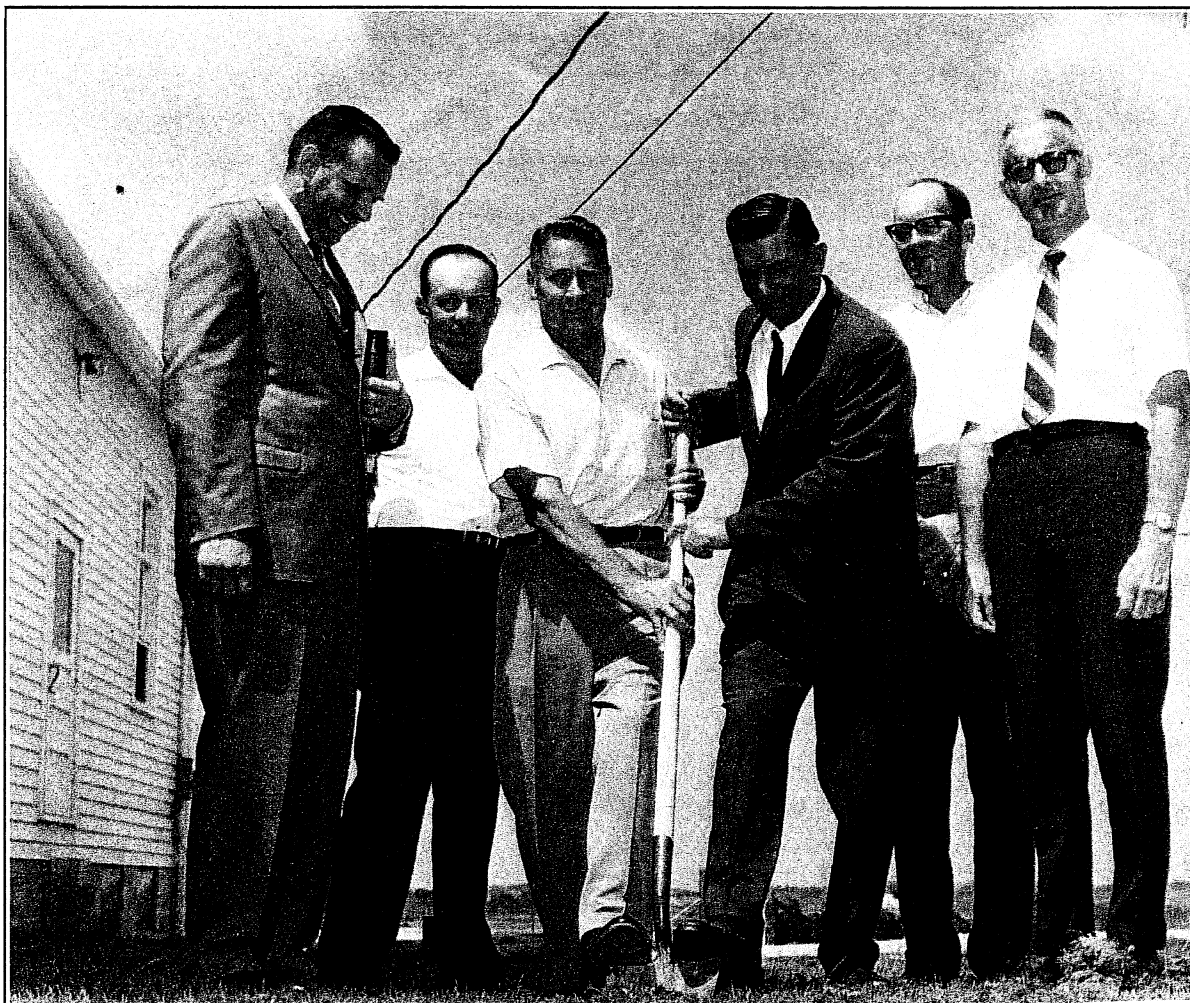
Groundbreaking for new addition on north side of the LaMoille Church
