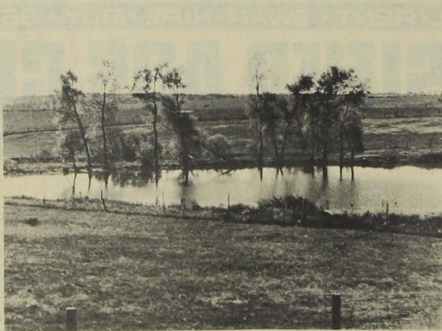
PONDS: Serious damage to the structure shown above has occurred long before the willow trees reach this size. The roots penetrate the fill and will cause leaks to develop. These unsightly trees
