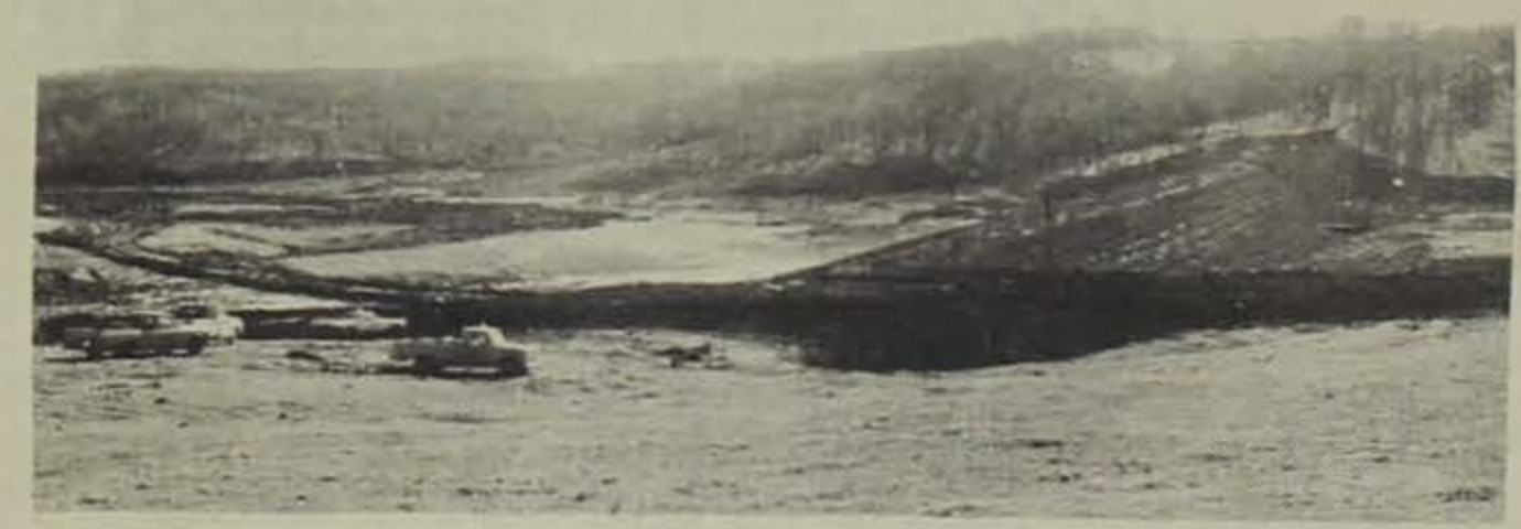
A soil conservation structure located two miles west and one mile south of Murray is shown shortly after it was completed in November of last year. The dam will create a 35-acre pond when filled. It is located on the Harold Pearson farm.
