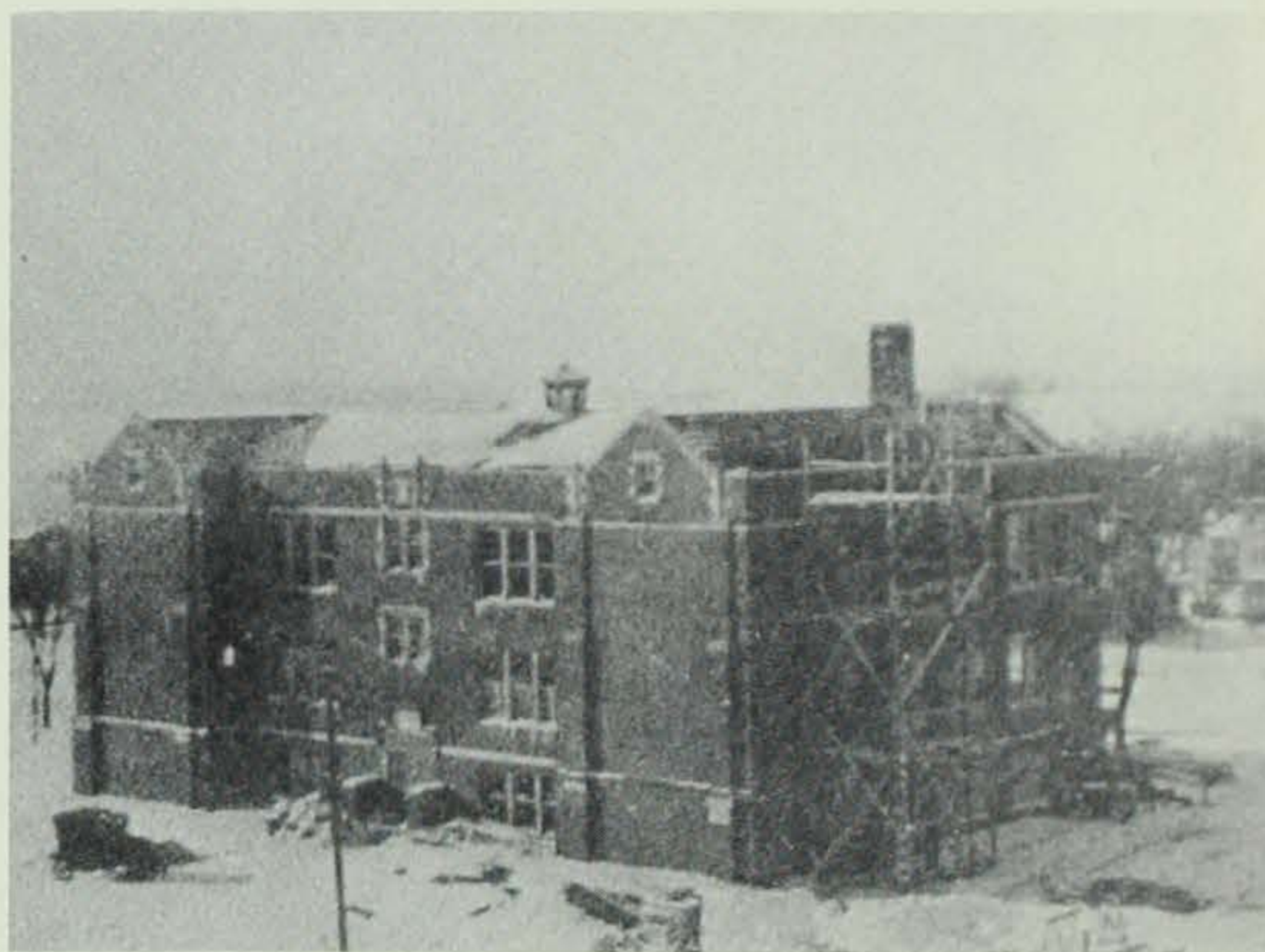
Erection of Smith Hall — 1925.
