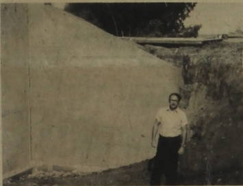
A COUNTY ENGINEER'S PART---Don Shaw, Ida County engineer, stands next to a reinforced concrete culvert on the Garfield Township road project. The slanted portion provides upstream gully stabilization. (Photo by Don Kauffman)
