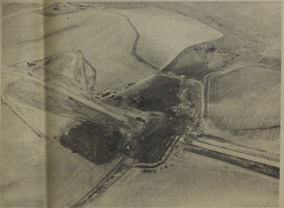
BUILDING FOR TOMORROW --Ida County's Crawford Creek Watershed has been one of the big projects highlighting the year of soil conservation in 1976. The aerial view shows work proceeding on one of the first structures to be built this past spring and located on the Marvin Krayenhagen and Stuart Lee property in Garfield Township south of Battle Creek. The structure, which cost about $50,000, has an 18-inch pipe running through it and will create a 5.8-acre permanent pool. (Photo by Aerial Courtesy of GOMACO)
