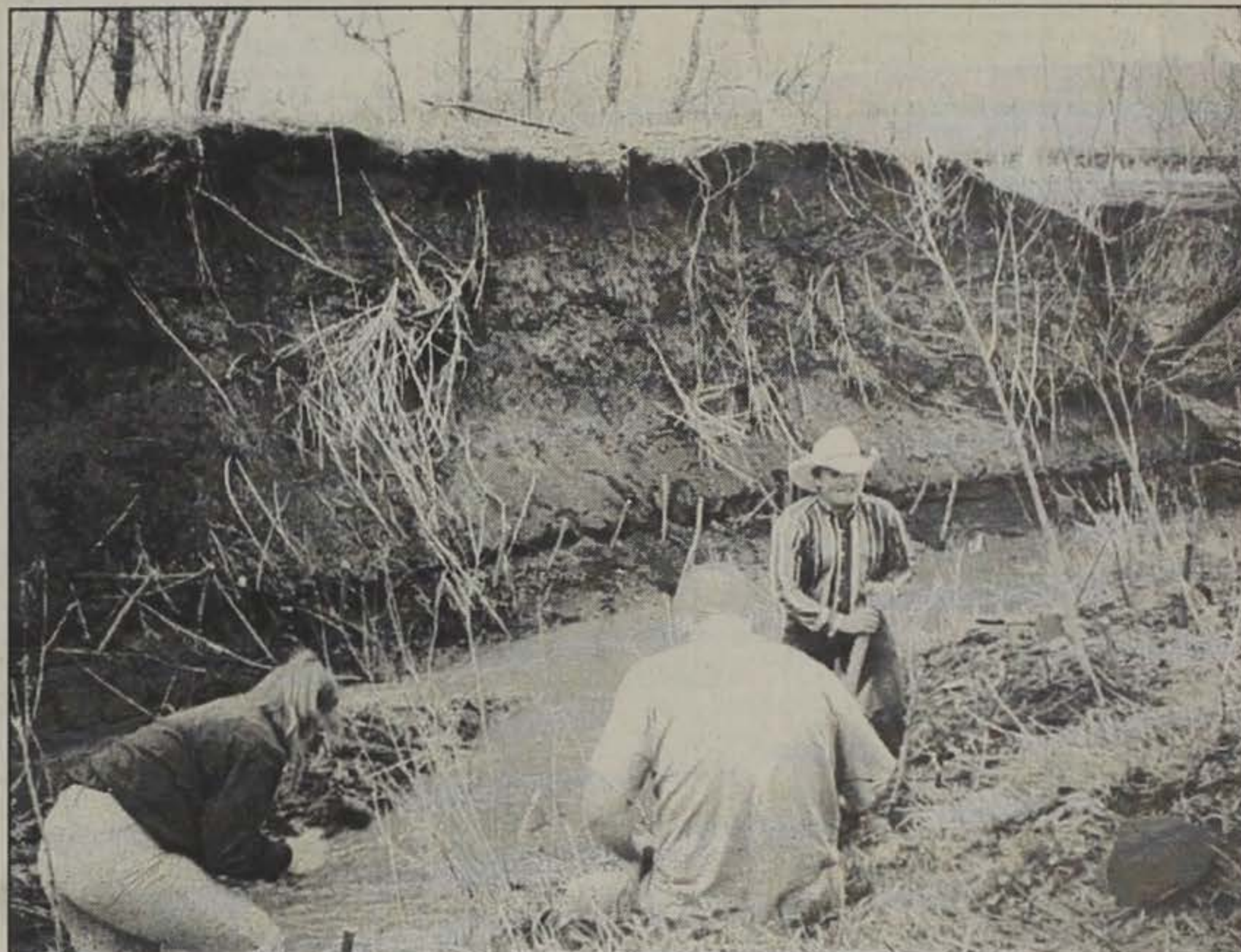
Murray students working on stream bank stabilization project.
