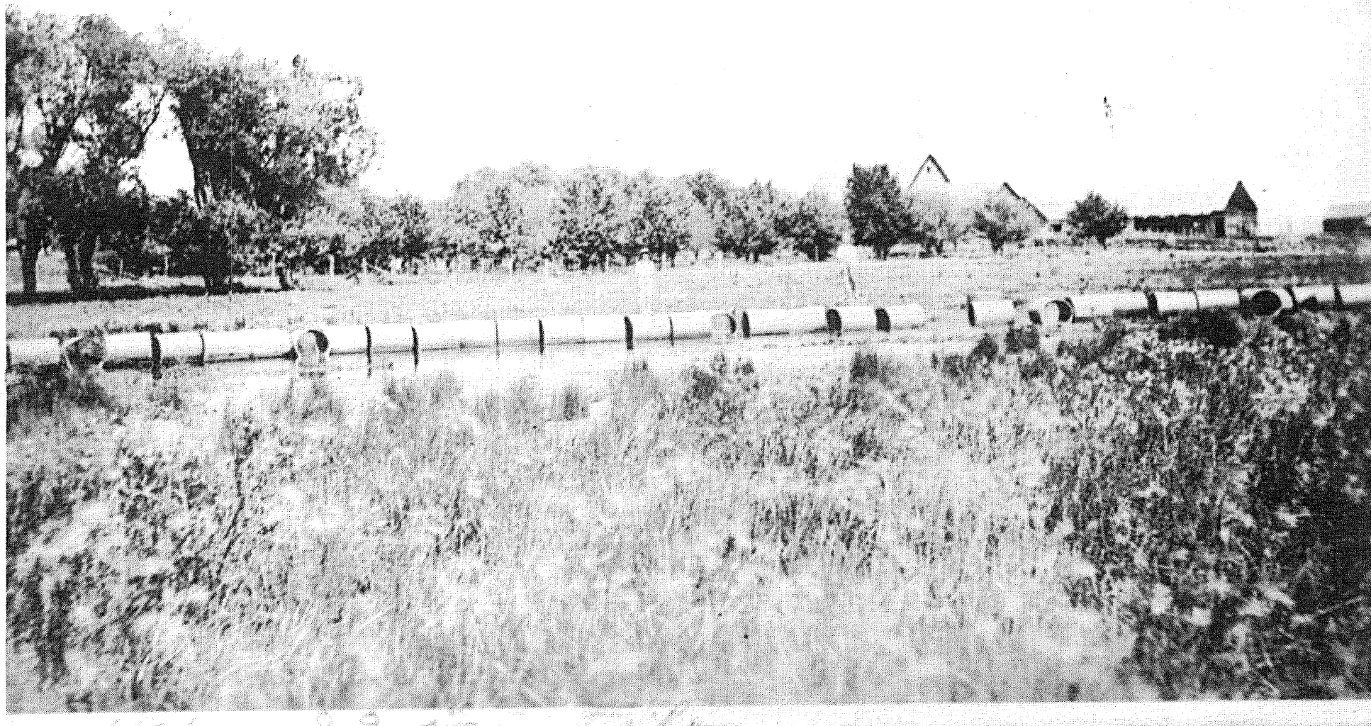
22 inch drainage tile. J.B. Crim Farm in northern Boone Co. 1918
