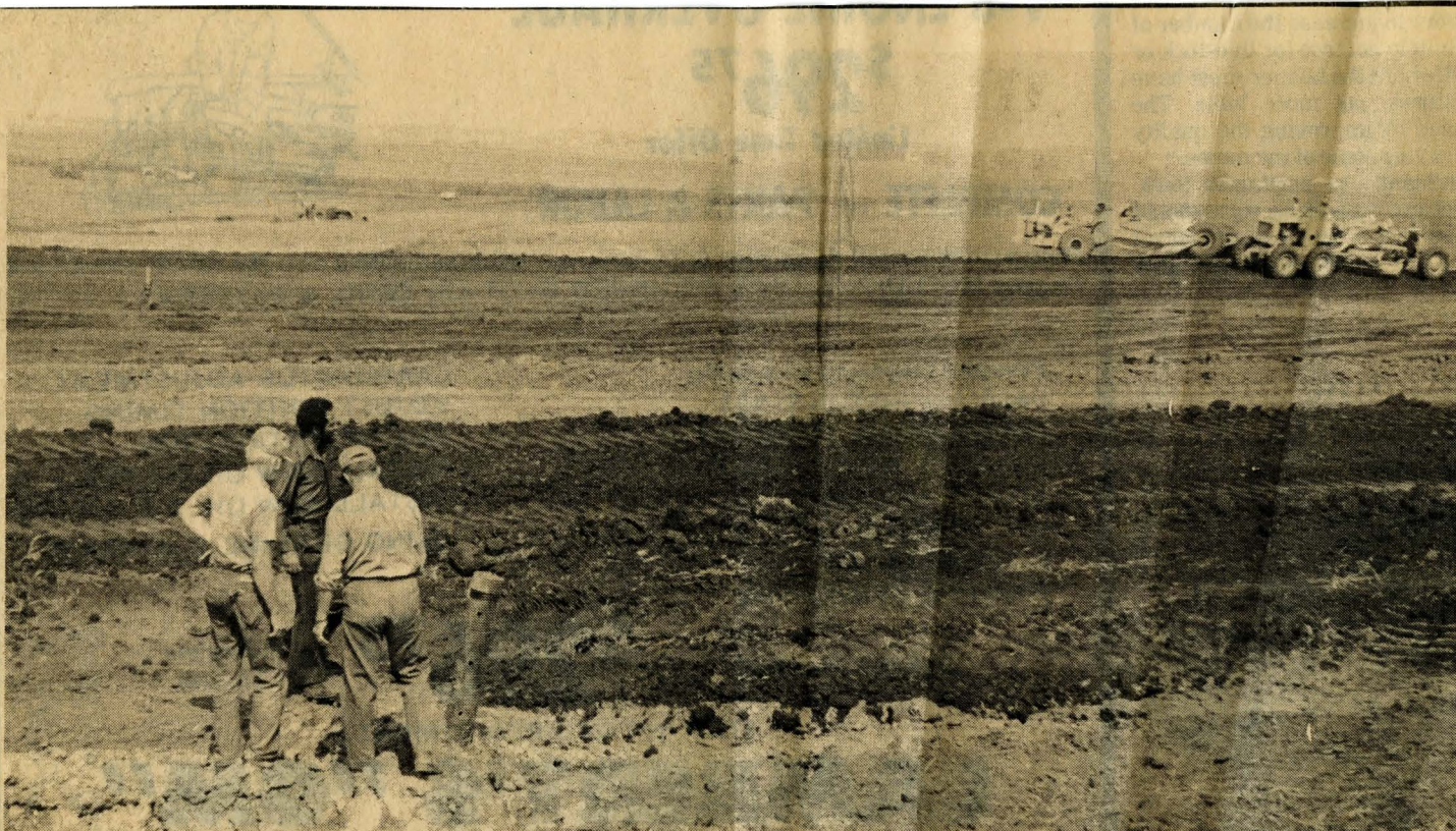
NEW TERRACES — William Baugh (center), conservation technician with the Fayette County Soil Conservation Service, visits with heavy equipment operators during the construction of new broad-base terraces on the Carl and Larry Recker farm northeast of
