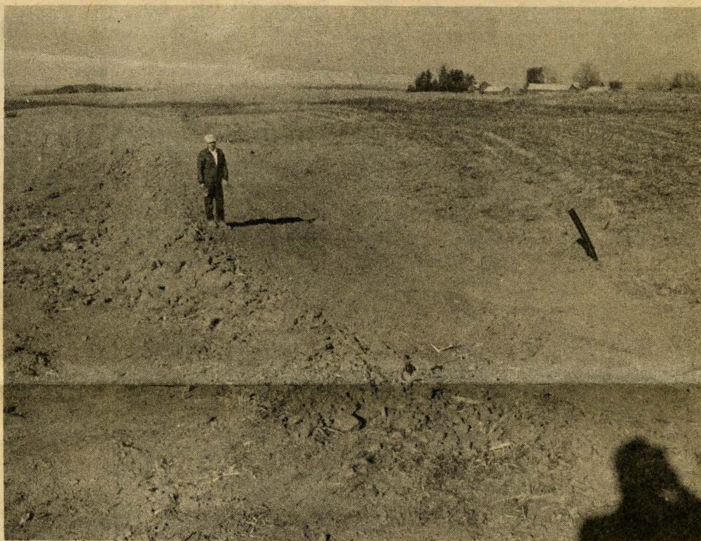
DRAIN PIPE at right will carry excess water from above the terrace on which Mr. McMillan stands, into sub-surface tile.
