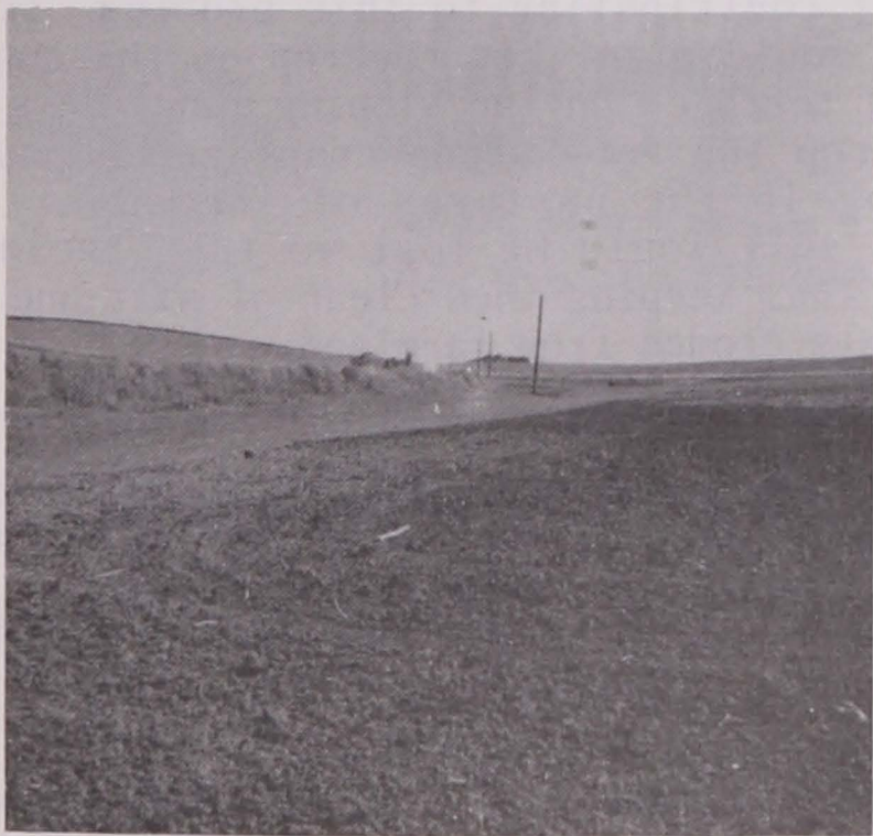
After tile were installed, the ditch was shaped into a sod waterway on the Coffman farm.
