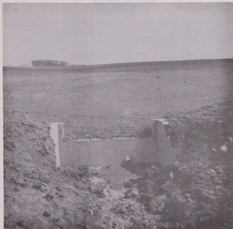
Completed structure on Mussig Farm. This structure controls the outlet of a sod waterway and provides a good tile outlet.
