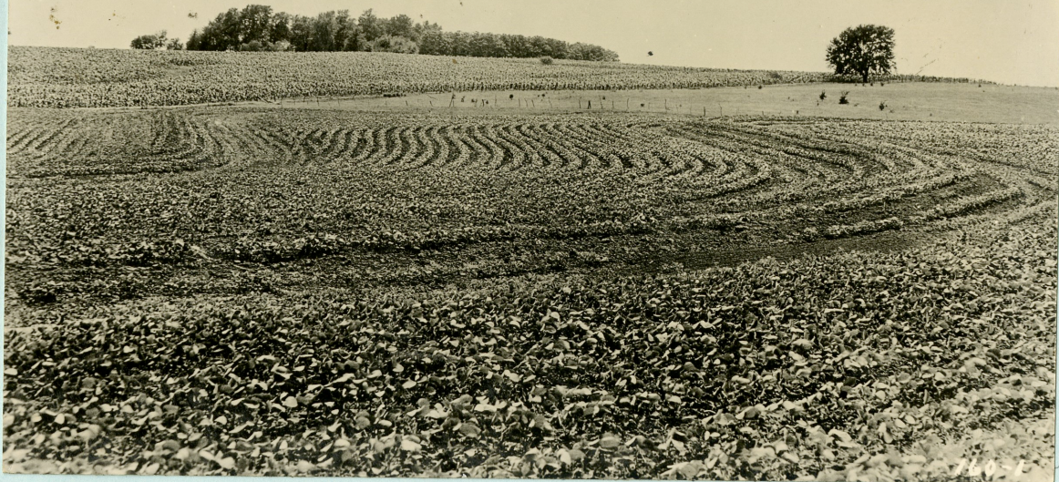
Contour farming on terraced fields, or planting crops on the level, will hold soil in place between terraces and conserve moisture for plant growth
