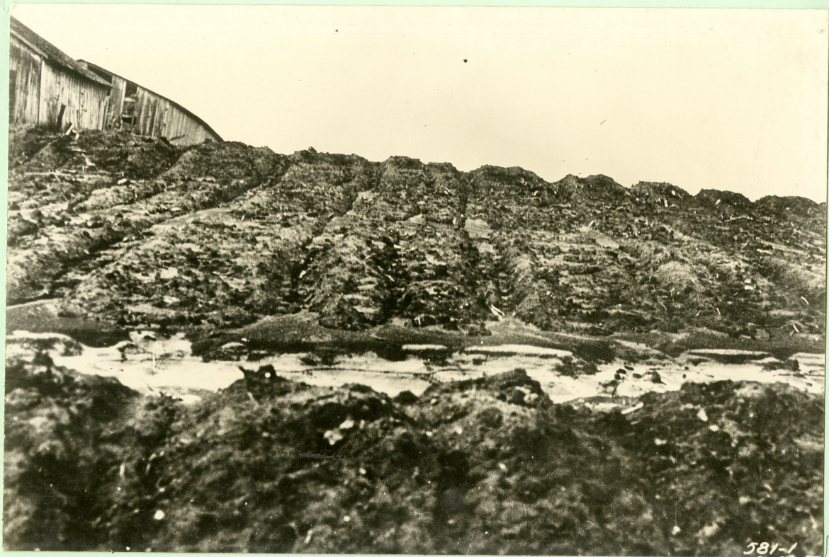
planting rows straight across these terraces is destroying the ridge of the upper terraces and filling the channel of the lower terraces with silt.
