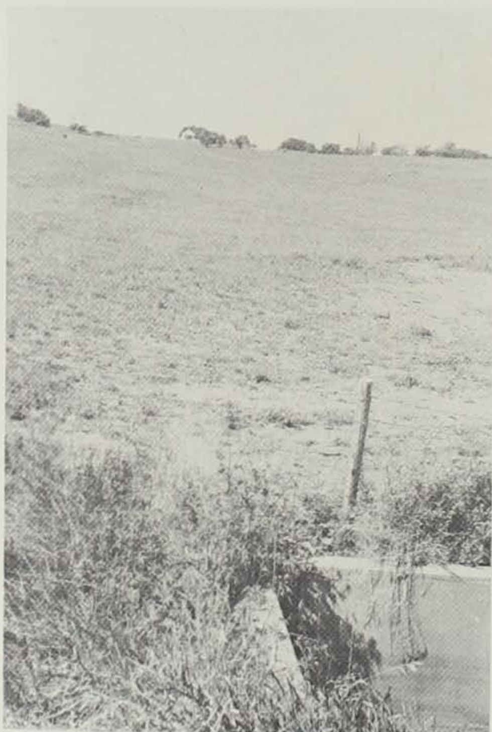
After Picture: Structural Water- way, Big Wyacondah Site 27-H-6 Lee Shelton Farm — SCS Photo
