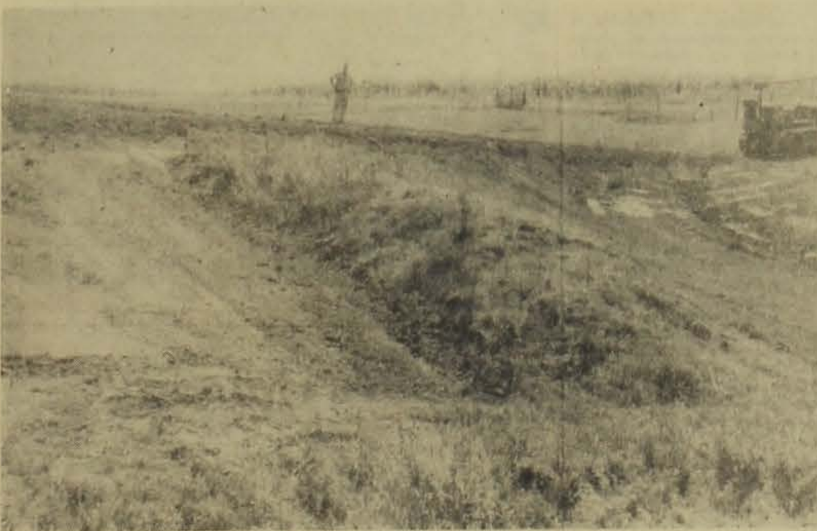
Here, in the making, is a diversion dike on the Pat Carbin farm. The bulldozer has been used to fill in the gullies that were on this hillside. The diversion dike on which Carbin is standing has been built up and the water will be diverted around the dike, until the sod has been established on the flume below. This flume, now shown under construction, will carry the water later, as the top of the diversion dike will be sliced off in order to allow the flume to carry the water away.
