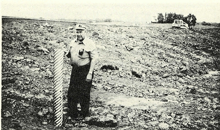
Clarence Beyer examining an inlet on a tile outlet terrace system during construction.
