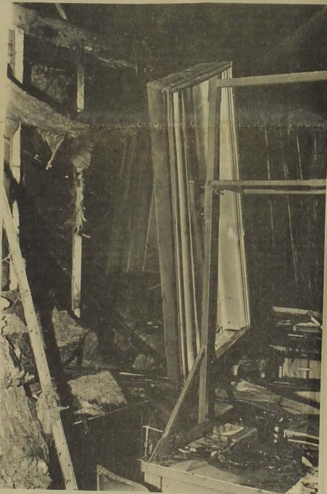
Ceiling meets the floor
