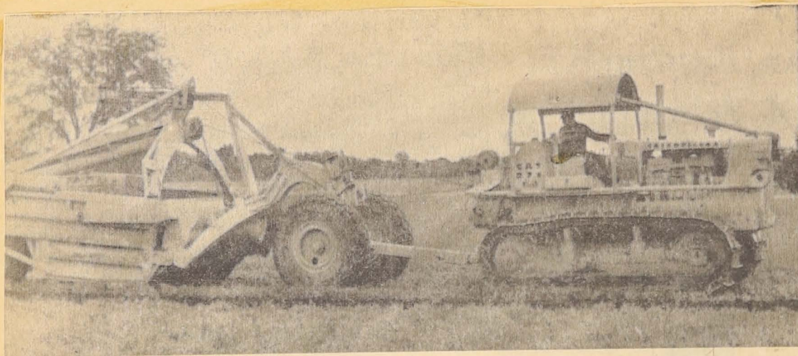
TERRACING is done by scraping earth from the high side of a field and filling in the waterways on the low side. Frank Woodall is running this earth mover for Leigh Raetz.
