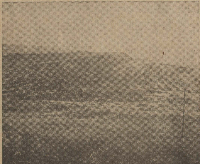
Grassed backslope terraces are being built in the 4,510 acre North Pigeon watershed north of Crescent. The work plan has been completed and approved by the local sponsoring group. It is now in Washington awaiting action by the Bureau of the Budget.
