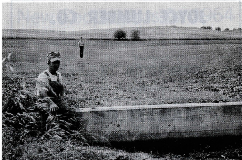
Concrete toe-wall structure with grass waterway above. Jerry Cranston, 3 miles south-east of Deep River.
