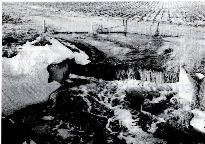
Re-inforced concrete structure controls overfall on the late Fred Bissett farm, 5 miles south-east of Montezuma.
