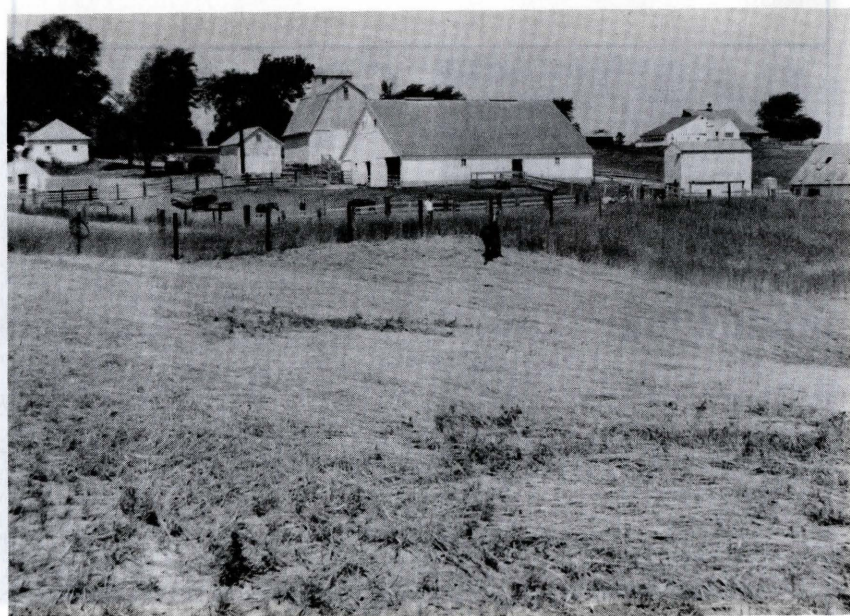
After: Photo showing lane on dam across 25 foot gully. Structure consists of 8000 cubic yards of earth fill and metal pipe outlet.
