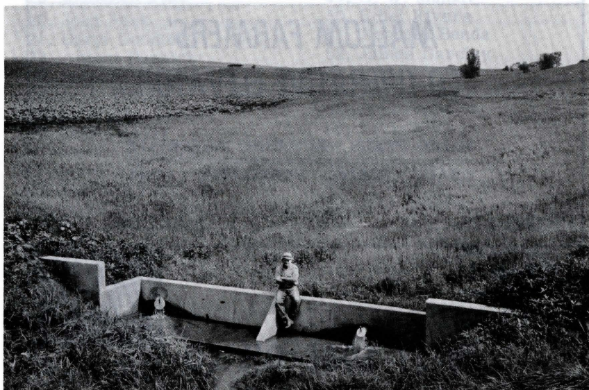
A 24-foot toe-wall structure on the Hugh Dillon farm, 4 miles north-east of Brooklyn. This structure stabilizes a waterway and provides an outlet for two tile lines.
