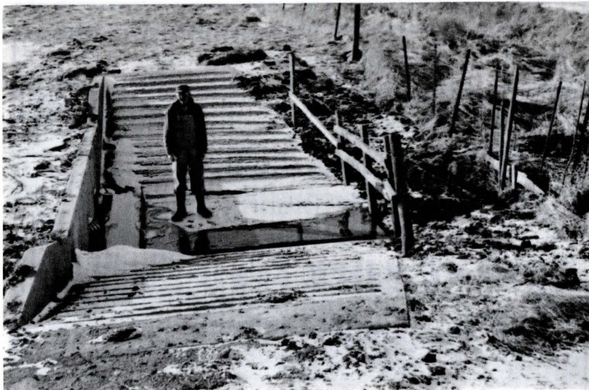
Triple-purpose ramp-type structure on the Milo Leimberer farm, 2 miles north of Hartwick. Structure provides, gully control tile outlet, and livestock water supply.
