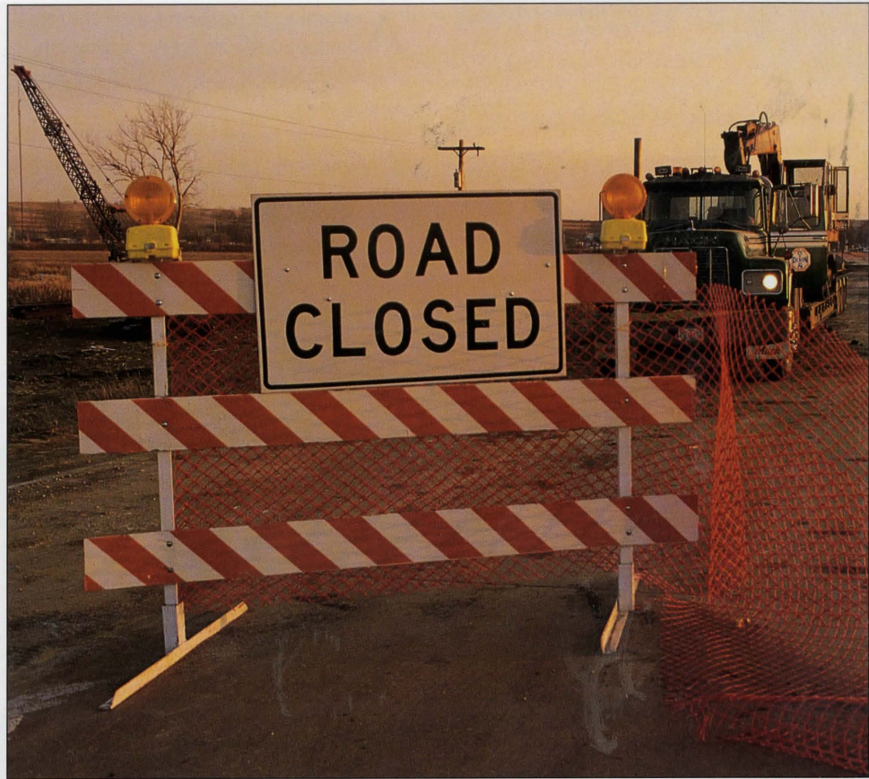
Many roads and bridges across the state, including this one in Montgomery County, were temporarily closed because of high waters or damages caused by flooding. 3
