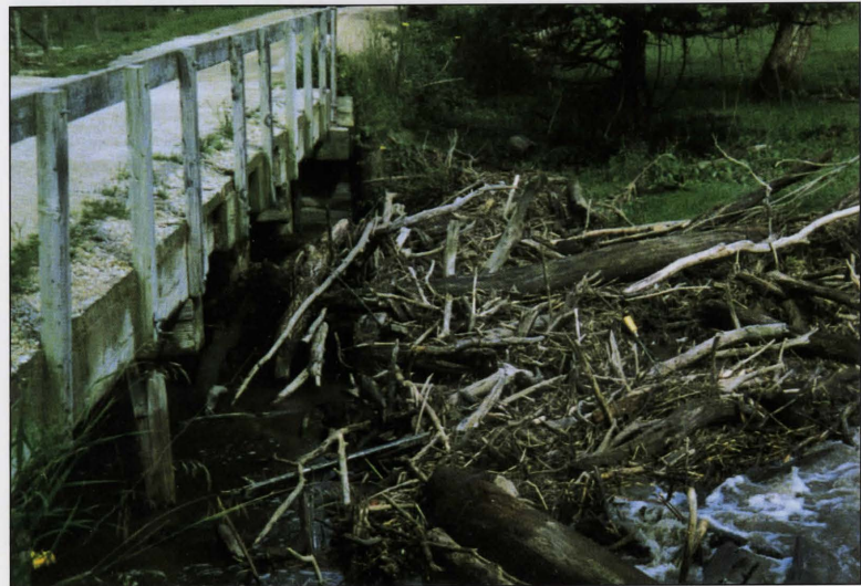
Debris removal projects, like this one in Howard County, were high priority EWP projects.
