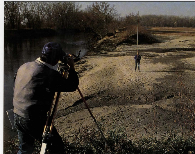
Randy Robb, Fremont County District Conservationist, surveys a levee repair project before it was completed late last fall.
