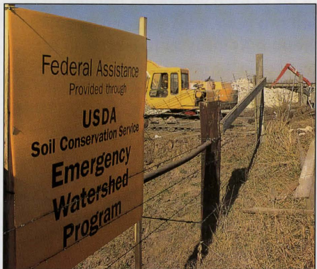
Many projects, similar to this Page County bank stabilization project, were funded through EWP.
