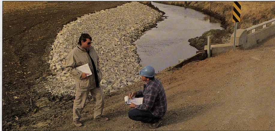
A bank stabilization project in Carroll County prevented this bridge from collapsing.
