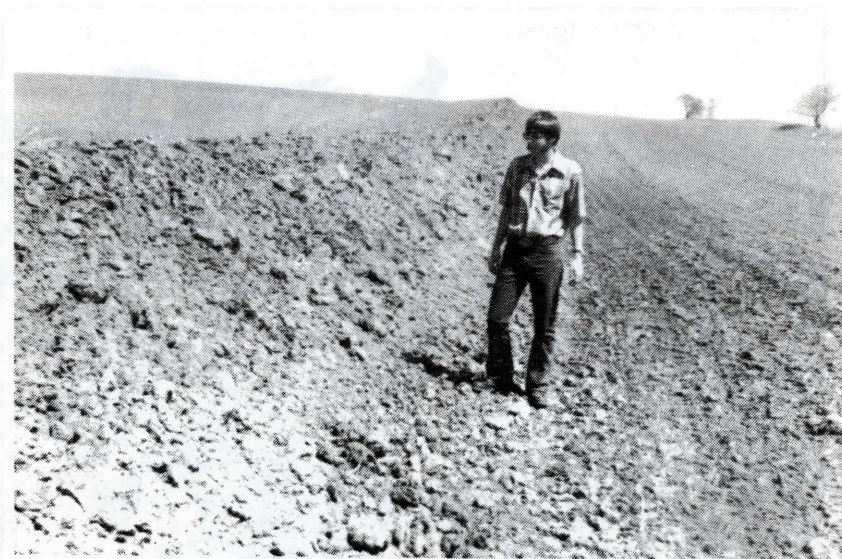
Mike Rich, Trainee, inspecting sediment basins installed on the Chief Alfa farm.
