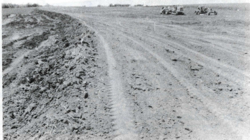
Basins under construction on the Raffety Farms.
