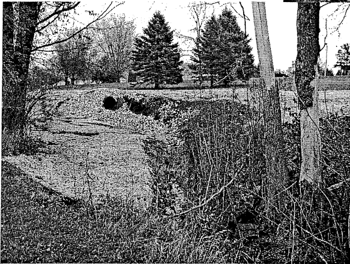
New Storm Sewer outlet fall 2003
