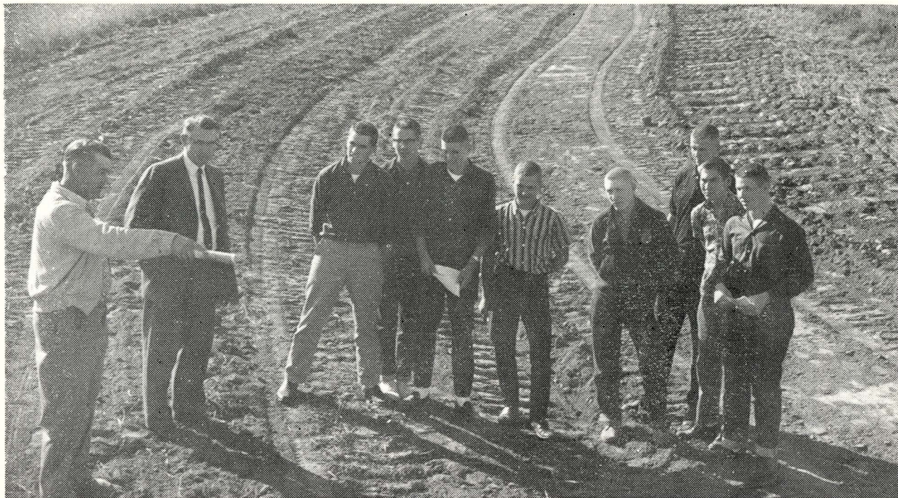
Clarence Beyer talking to Ralph Gruenwald, Tipton, and his Ag class about the terrace under construction on the Gruenwald farm.
