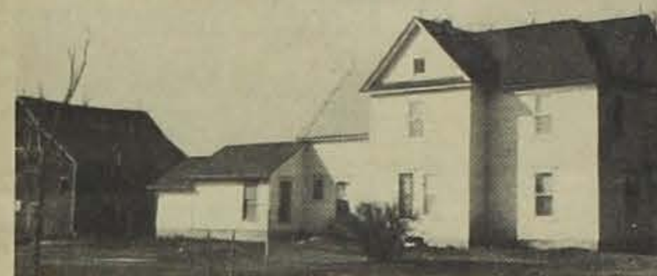
East of the Jesses is this large old-style country home on land they rent, which is occupied by the D. Minard family. This was the home of the late Charles Rupprichs.
