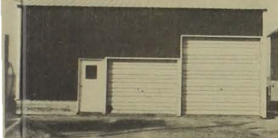
The steel building was erected on the Jesse farm last fall. They farm approximately 600 acres.
