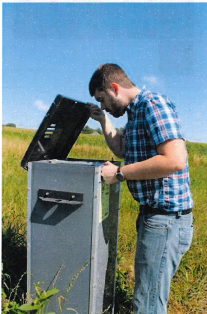
Shane Wulf, Miller Creek Watershed project coordinator, looks into the water control structure at the edge of a denitrification bioreactor south of Waterloo.
