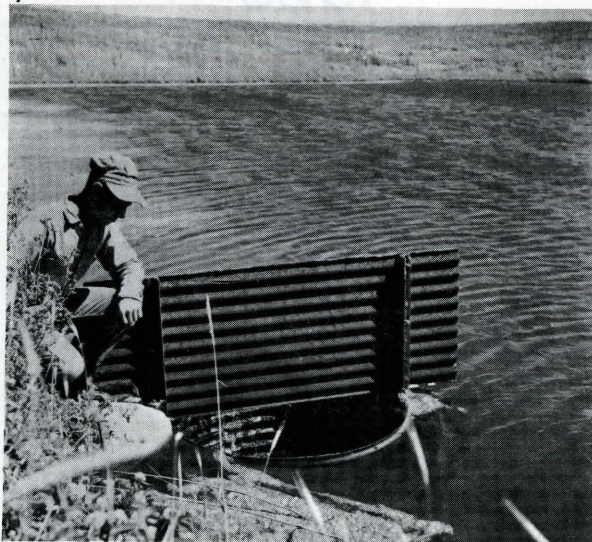
William Nagel Jr. inspects anti-swell baffle and drop pipe on the Nagel farm, Grinnell. The asphalt coated culvert pipe allows flood water to flow down and through the earth dam.
