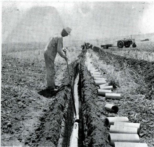
David Anthony places tile in a new tile ditch already flowing with water. All tiling contractors were more than busy in 1959.
