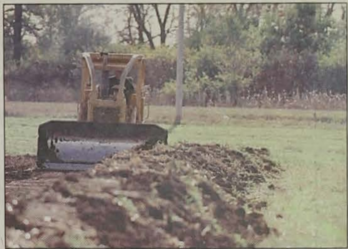
BRANDON POLLOCK / Courier Staff Photographer With crops out of the field this fall, Dan Schmitz built terraces in some fields at Laurel Ridge. The earthen terraces break a long slope into shorter sections so rainwater never builds up enough speed to cause gullies.
