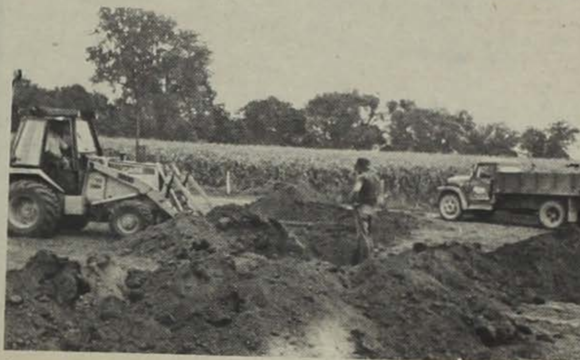
In moves the equipment and the project begins.
