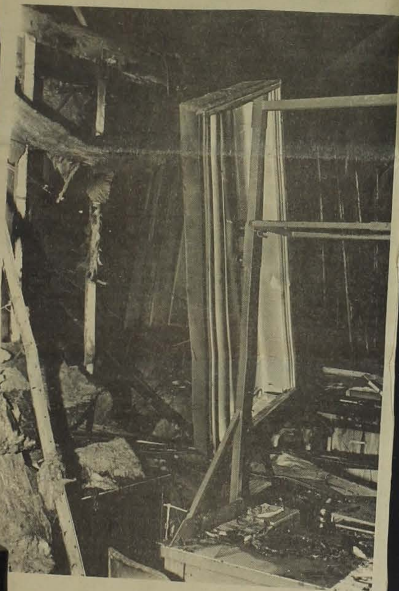
Ceiling meets the floor
