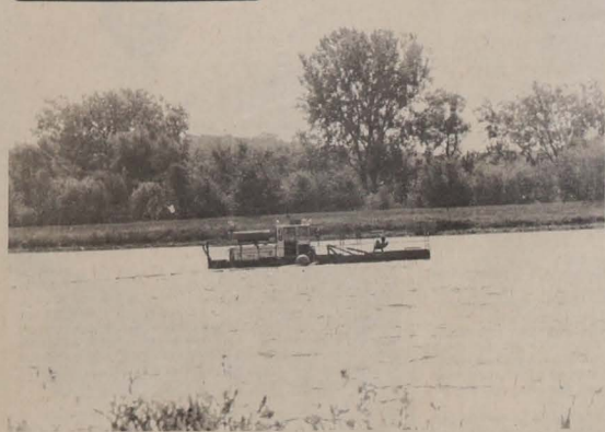
The dredge operating on Union Grove Lake this summer has begun pumping out silt, after area farmers altered their land use practices to prevent further erosion.
