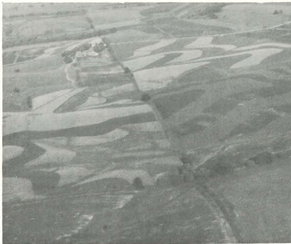
Stripcropping on the Virgil Meyer and Herbert Swain farms in York Township. Stripcropping gives better erosion control than just contouring.
