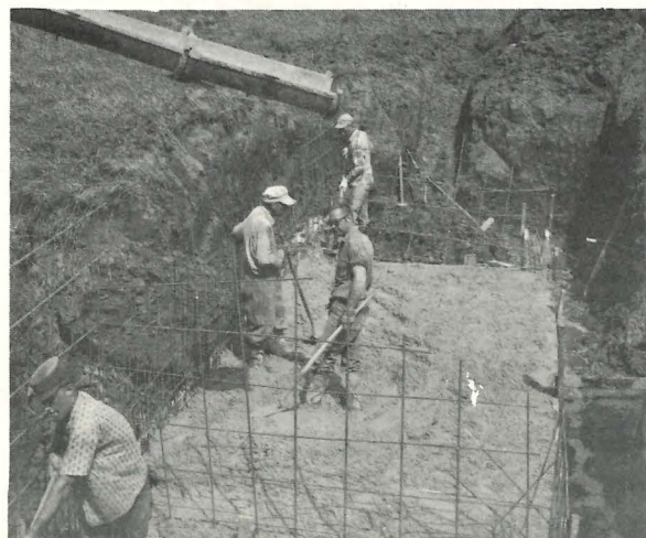
Reinforcing steel is in place and concrete being poured for Joe Black's structure. After the structure was finished by Ron Ahrens of Harper and his crew a waterway was constructed to replace the ditch shown in the top picture.
