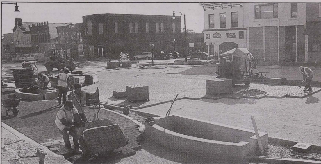
The installation of porous pavers north of the Elm and Vine intersection in West Union began in September 2012. (Mike Van Sickle photo)
