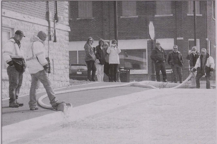
As state and local officials observed in April 2012, West Union Utilities Department employees (foreground, l-r) Andy Larson, Scott Johansen, and (at fire hydrant) Mike Moser demonstrated the speed in which the porous pavers in the Green Pilot Streetscape Project absorb water. (Mike Van Sickle photo)
