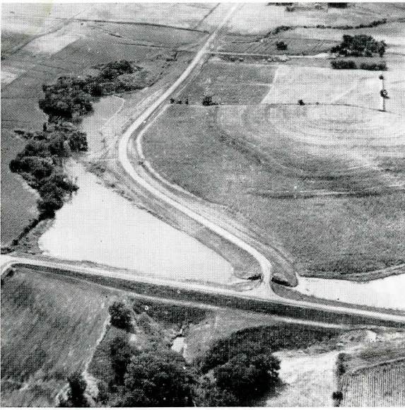
Looking west from Conaway dam, relocated road and concrete flume at upper center of photo. This structure built in cooperation with Mills County Supervisors.
