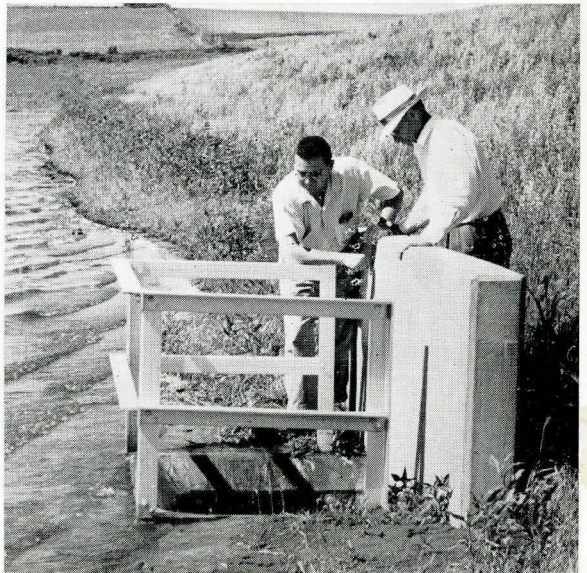
Troy Rhody, County Engineer, and Wm. Van Orsdel, chairman of County Supervisors, check the inlet structure of dam on Timmons farm.
