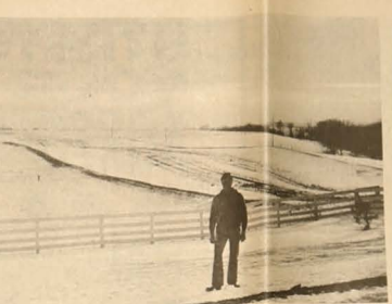
RUNOFF FROM neighboring fields and a highway were causing erosion problems on the Kenneth farm in West Union. Terraces and surface ditches were installed to control the water. The terraces were constructed parallel to the road to maintain good fertility of the field. A terrace below the terraces was also built by the work.
