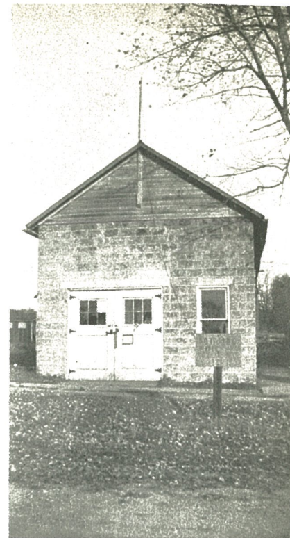
Town Hall and Fire Dept.
