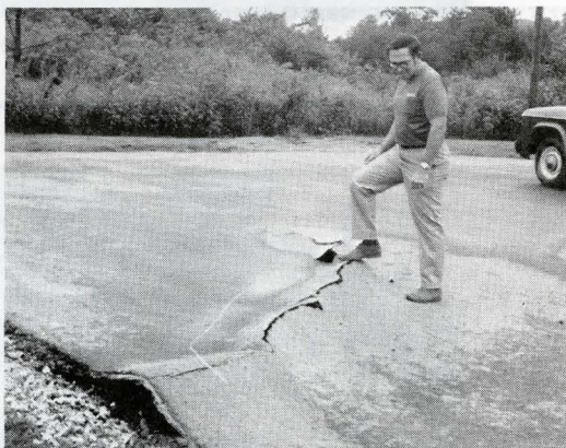
Harry Bryant takes a look at damage done to a black topped parking lot after an earth slide caused by the long rainy spell. Oren Champ helps Harry check the depth of earth slippage, which later slid several feet farther causing Division Street to be closed for extensive repairs. Soil information can be highly useful to city land users to help avoid such problems before they occur.
