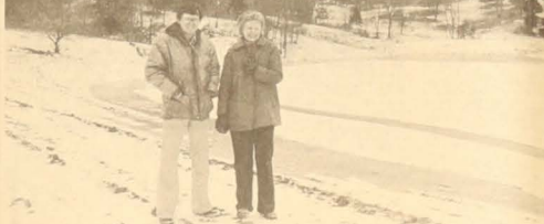
THIS GRADE stabilization structure was completed during November 1979 and is located one mile south of Wadena, standing on the dam is landowner Jean Savage and District Conservationist Jerry Muff. This structure
