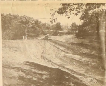
This impoundment grade stabilization structure (pond) recently finished in the watershed will eliminate gully erosion and stop 50 acres of sediment from reaching Pine Lakes.
