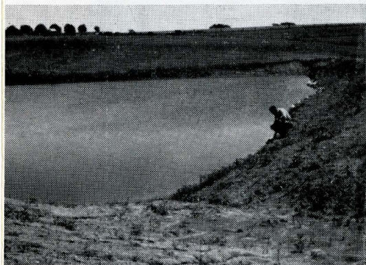
John Gordon pond, S.W. of Plano. Designed by SCS with cost sharing through ASC. It has 1\frac{3}{4} ac. of water at spillway elevation. The drainage area has been reduced from 45 to 30 ac. by diversion and terraces. Mr. Gordon gets 3.5 acre feet of flood retention by keeping the water surface 2\frac{1}{2} ft. below the twin sod spillways by letting the 2" livestock watering pipe run during the rainy periods. This gives him 1 acre of water, 18 ft. deep for livestock water, garden irrigation and plenty for neighbors who's wells have gone dry.
