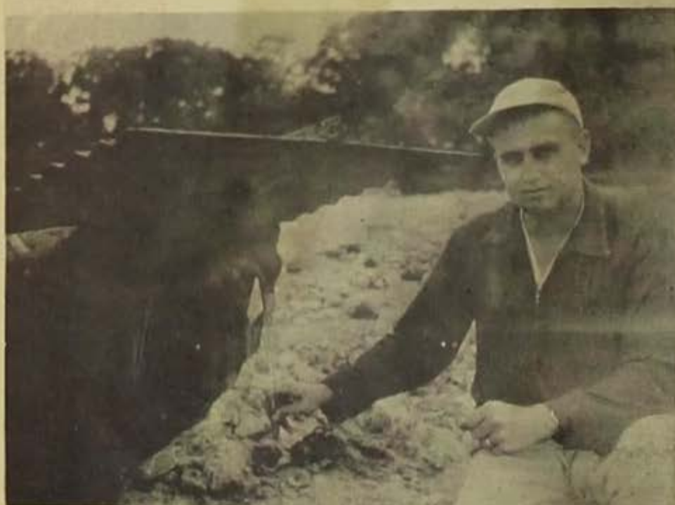
Cal Moore of the Hardin County Soil Conservation Service is shown at inlet of the 18" overflow pipe which is imbedded in the massive earthen dam. The picture above shows Cal Moore inspecting the outlet of the 18" overflow pipe at the lower end of the 40 to 50 ft. high earthen dam.
