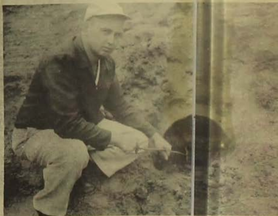
Cal Moore of the Hardin County Soil Conservation Service is shown at inlet of the 18" overflow pipe which is imbedded in the massive earthen dam. The picture above shows Cal Moore inspecting the outlet of the 18" overflow pipe at the lower end of the 40 to 50 ft. high earthen dam.
