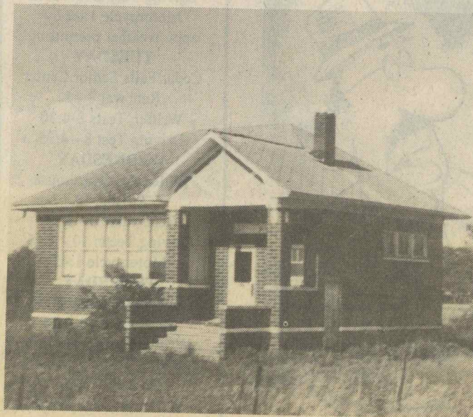
Norton Corners School House built in 1928.
